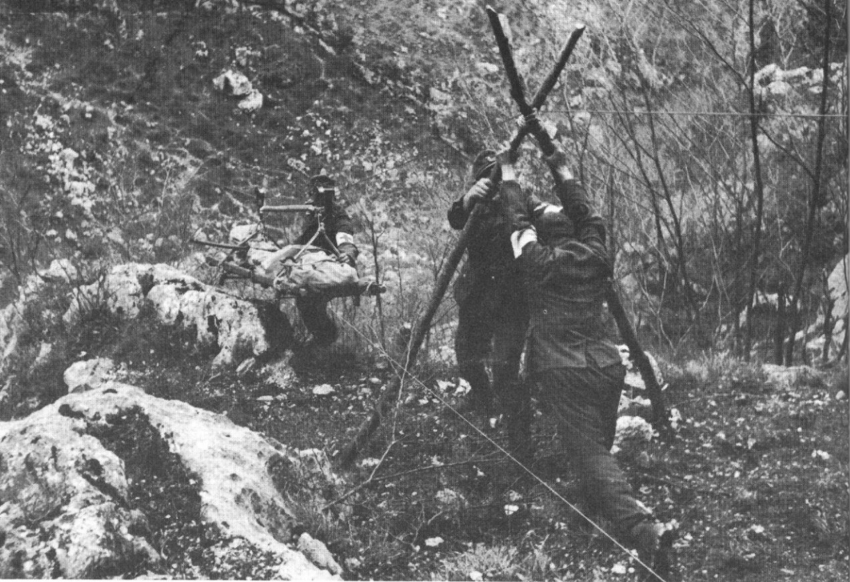
These pages and following two pages Mountain rescue. Man-handling a stretcher case down a vertical rock slope by means of lines secured from an overhead bipod and transferring the casualty to a two horse-power litter (313/1026/7, 13, 17, 22, 24 and 27, 313/1024/13 and 307/784/6).
